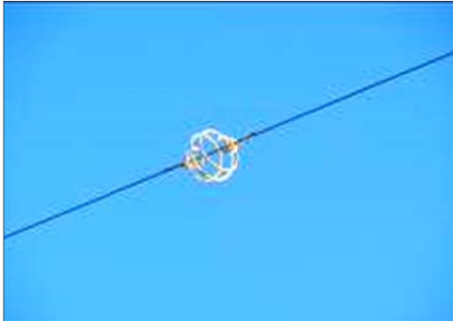
Photo 1 Bird diverter on the earthwire
